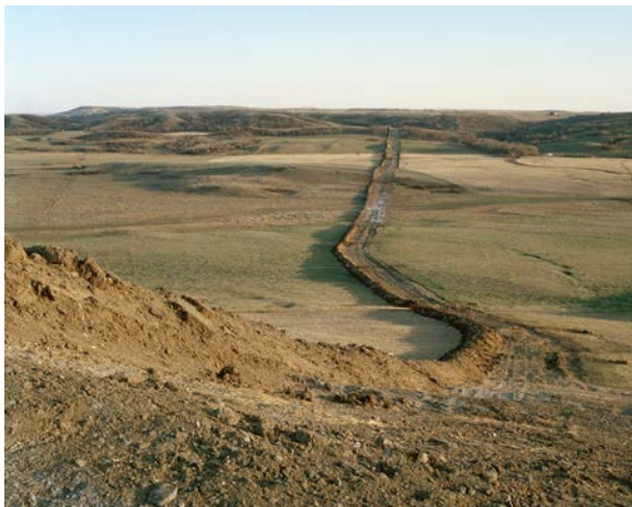
Pipeline constructed on land seized by eminent domain
